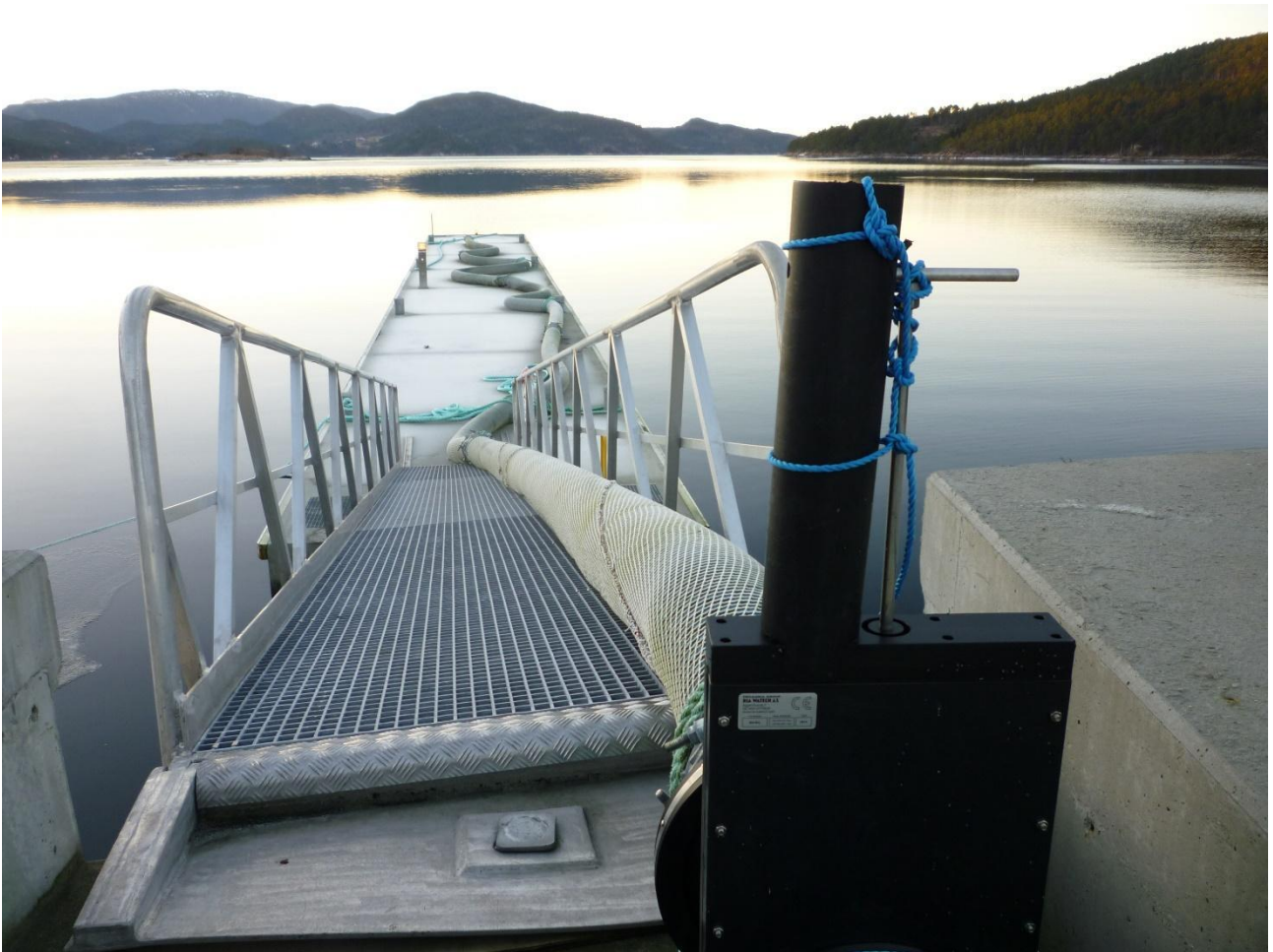
FIG 48. Transport pipeline for loading smolts aboard well boats.
