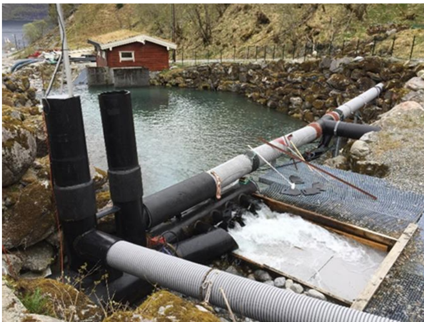
FIG 17. Built-up reservoir next to water intake from river.
